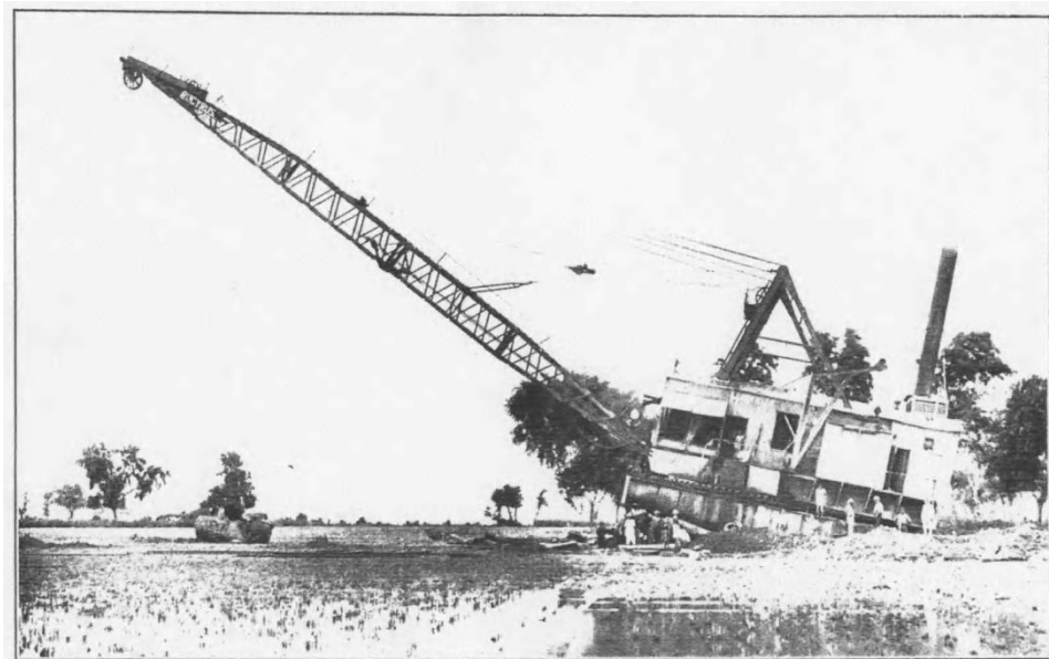
“Jacob Bahadur” excavator – general view showing the rear part of machine sunk in a dhoro near Pitpikar on the 24 th July 1929’, N.a., The Opening of The Lloyd Barrage and Canals , p.11.
