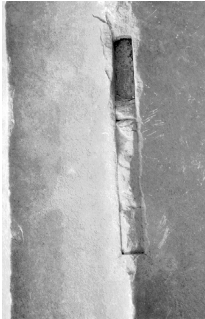
Fig. 9. Arris repair on block 809.
