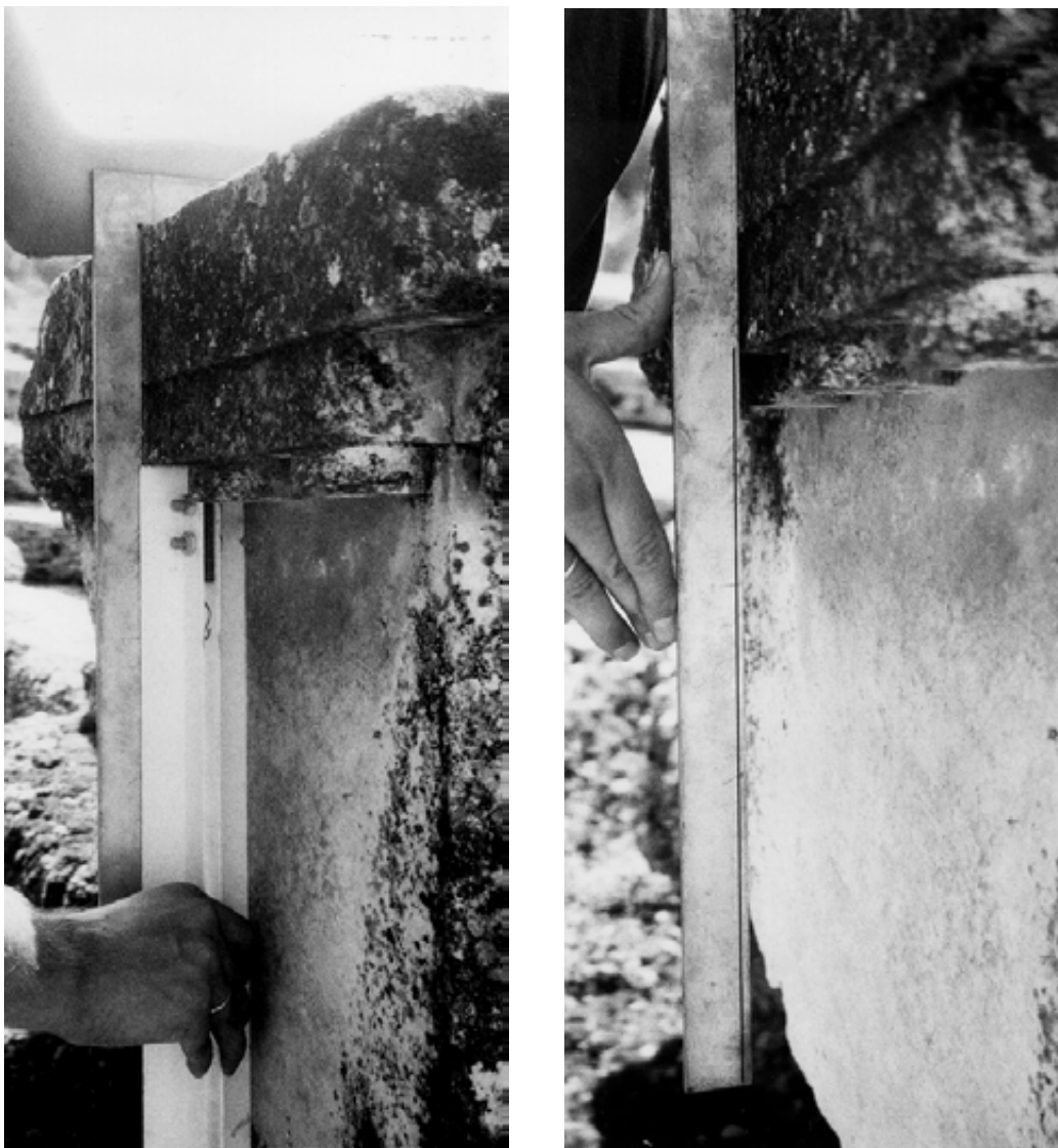
1. Architrave block, from corner. Measuring the angle. The line drawn on the metal square (right) enhanced. (Photographs by P. Pakkanen, 1995.)
