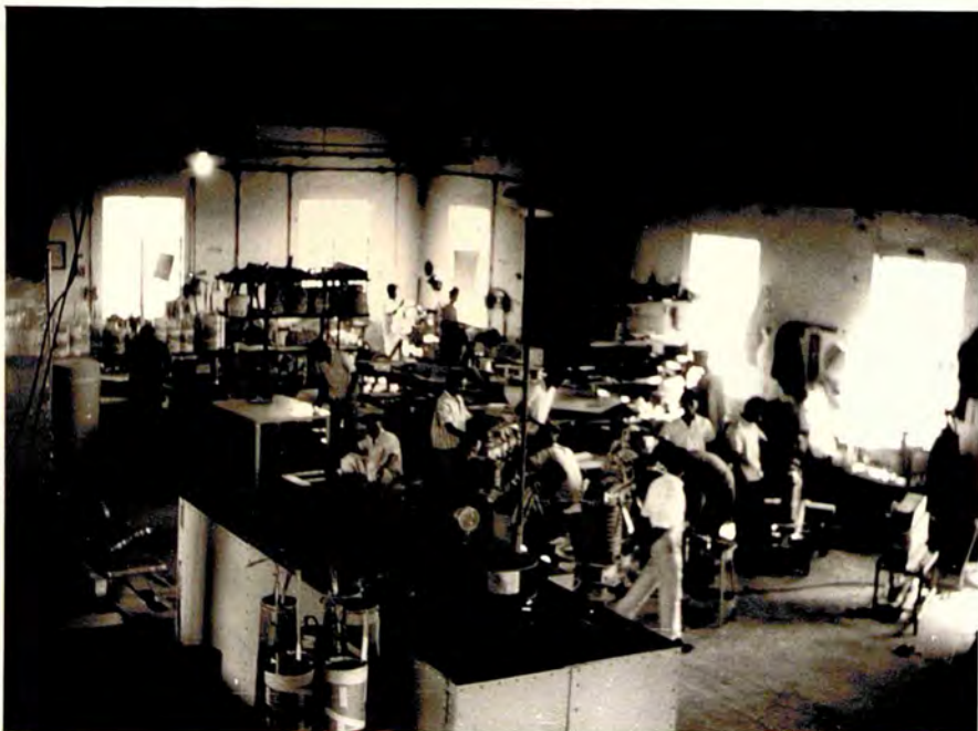
Plate XIII - Factory-floor of Electric Transformer, Sanathnagar.
