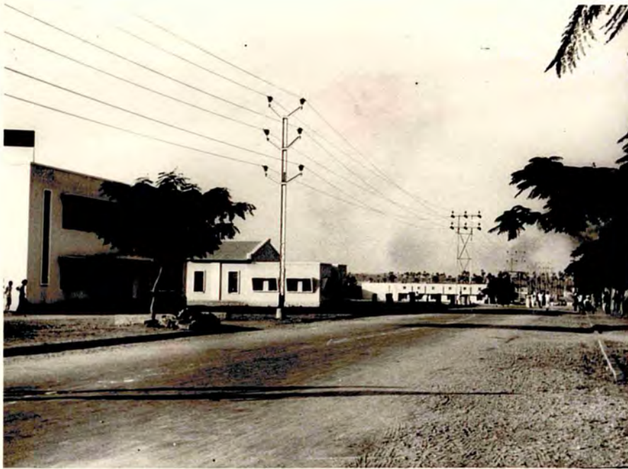
Plate X - State Bank of India and Raw Material Servicing Centre, industrial estate, Sanathnagar.
