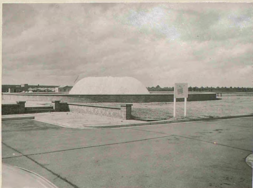
Plate I. An aeration basin fountain.
