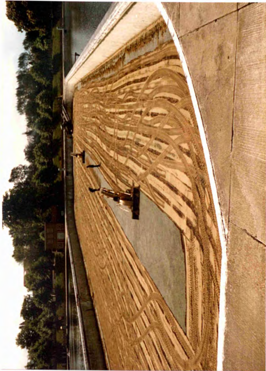
Plate 2.1 Cleaning of a slow sand filter bed by removing the surface inch of sand
