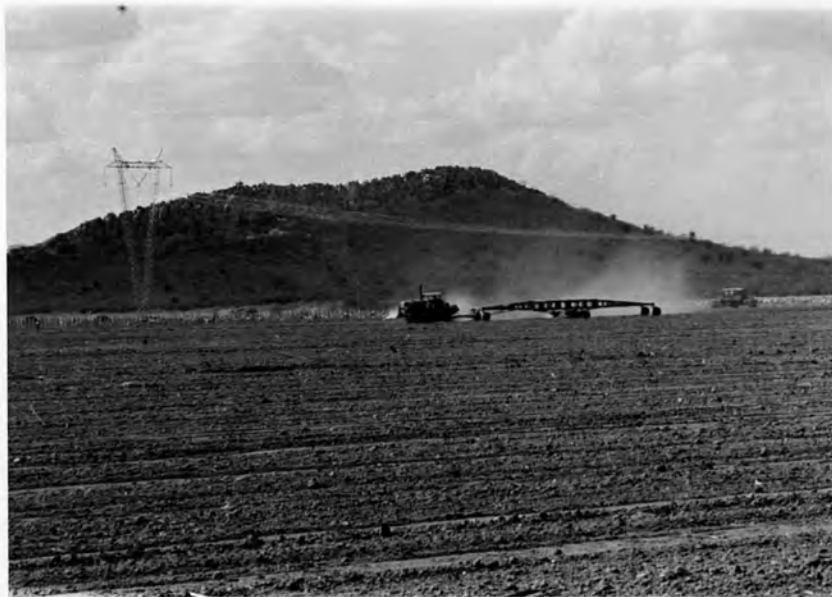
Plate 4. Earth moving equipment being used to level land on the capital-intensive CODEVASF Tourão project (Juazeiro County, 1981).
