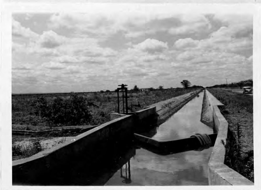
Plate 3. Irrigation system on the capital-intensive CODEVASF Bebedouro project. Main canal, siphons, sieve to secondary canal, fields in distance and unutilized areas in foreground (Petrolina County, 1981).
