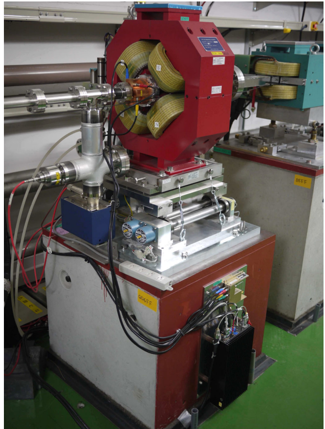
FIG. 8. Quadrupole magnet (QD6FF) and C-band CBPM assembly on a ATF2 mover. The rf processing electronics is mounted at the bottom of the concrete girder.
