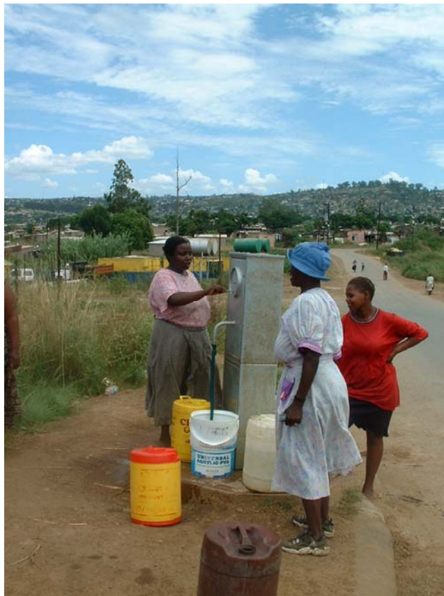
Figure 6: “Free Water” Standpipe in Bhambayi
