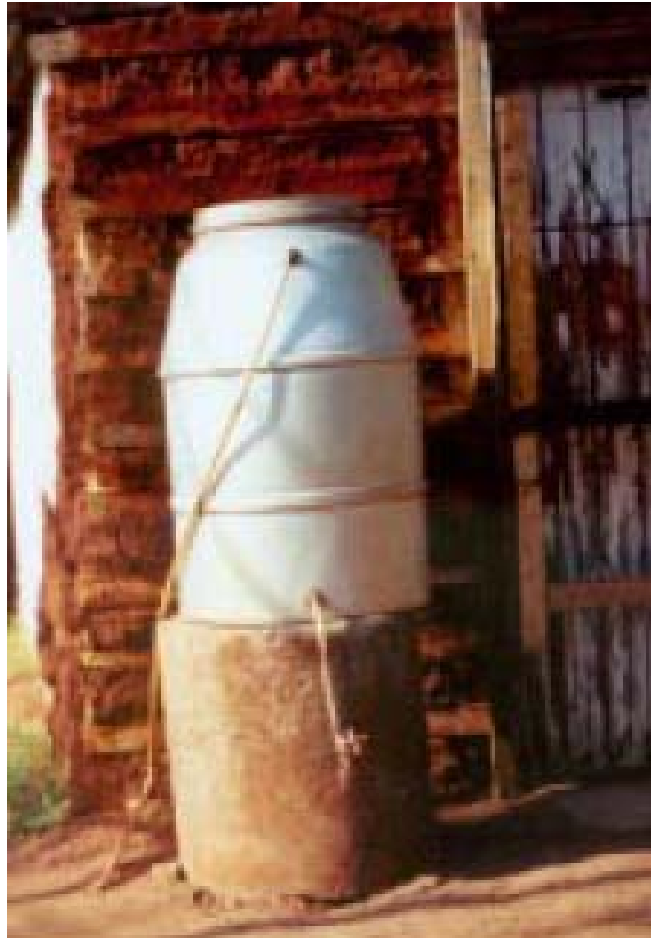
Figure 5: The Durban Ground Tank – a 200 litre tank of water, filling once daily
