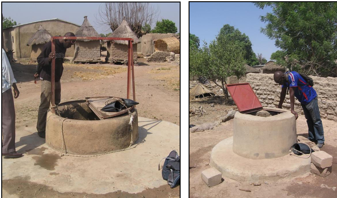
Figure 7.4. Examples of wells upgraded as part of the WaterAid self-supply pilot
